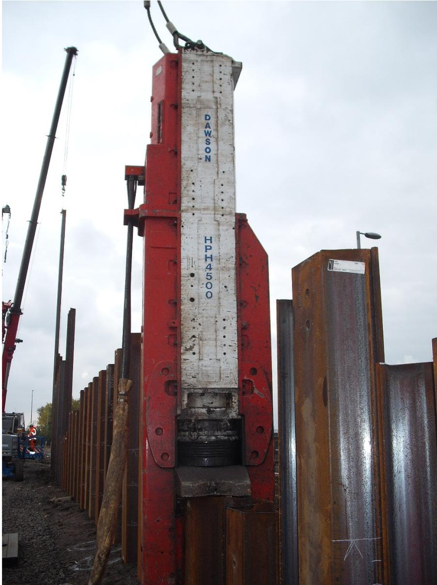
Figure 2 - Impact hammer in the field driving PU32<sup>+1</sup> sheet piles
